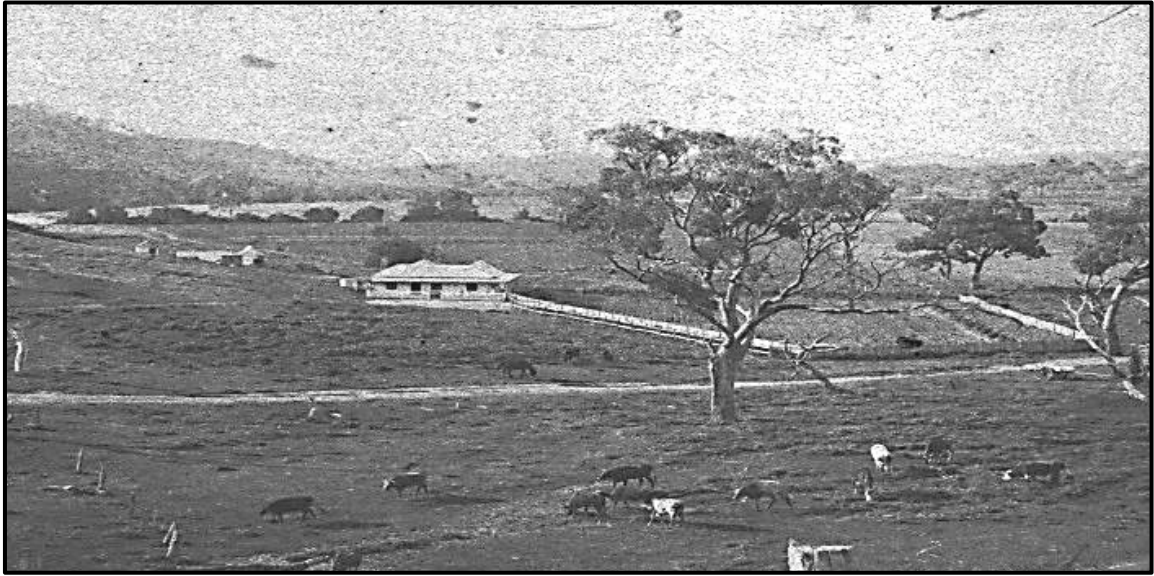
The homestead at Good Hope . Fifteen family members lived in this tiny bungalow; it was removed prior to the Burrinjuck Dam resumption.
